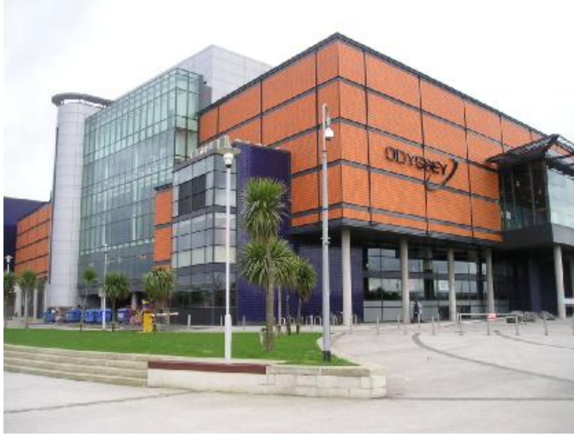
Fig.14. Photo of the Odyssey Pavilion millennium project.
