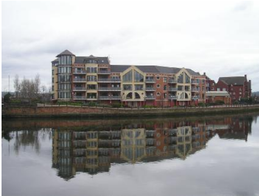
Fig.12. Photo of riverside apartments.
