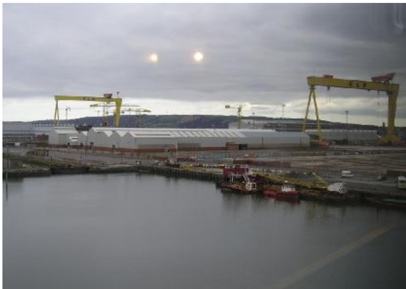
Fig.45. Photo of Titanic Quarter site today, looking towards the cranes of the Harland and Wolff Shipyard.
