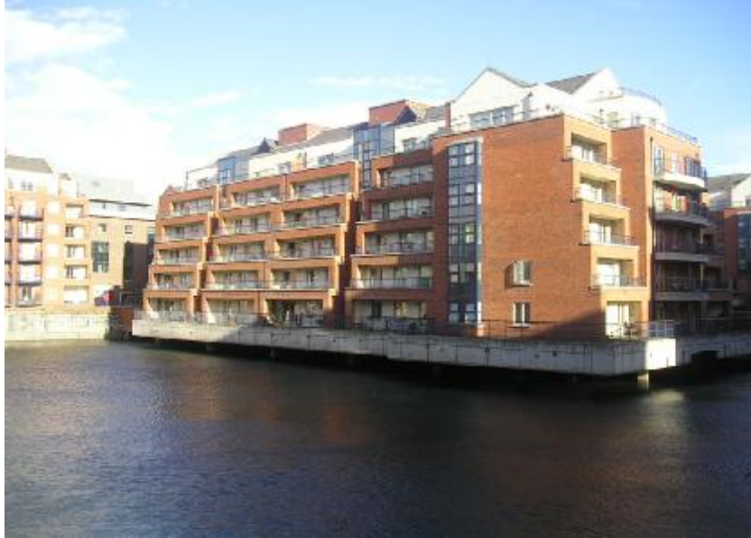
Fig.21. Photo of new apartments located in Georges Dock.
