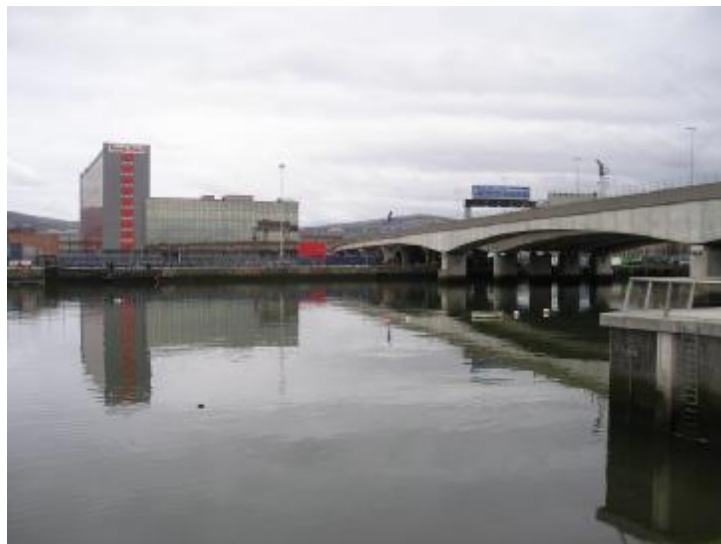
Fig.6. Photo of the Cross Harbour Bridge.
