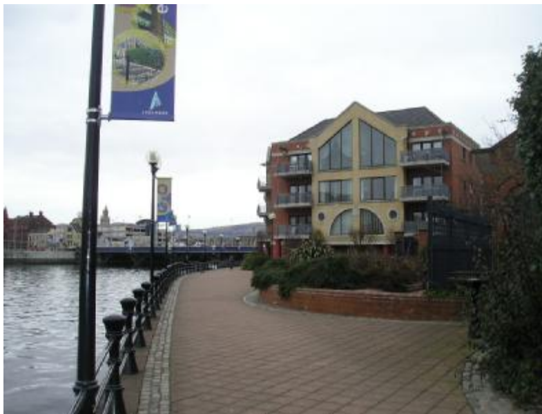
Fig.8. New Apartment living opposite the Waterfront Hall.
