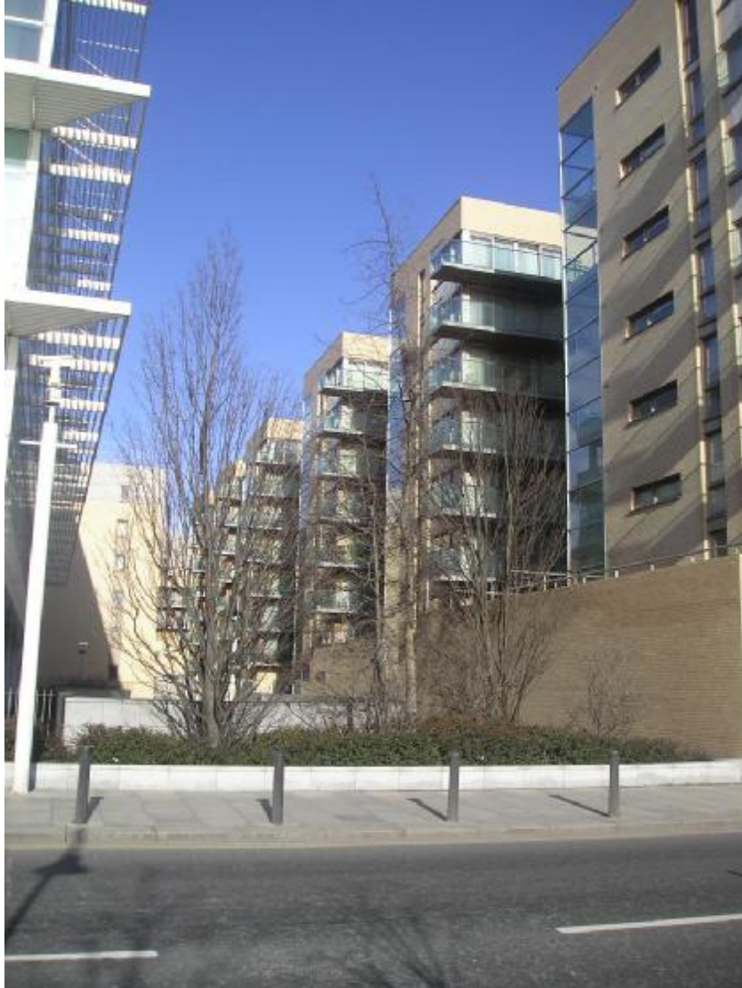
Fig.22. Photo of new apartments at Clarion Quay development.
